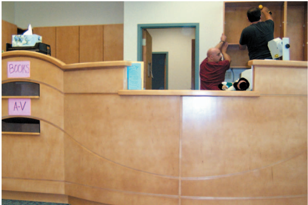
Walbridge plans to do more high-end millwork for libraries, schools and health care customers.
